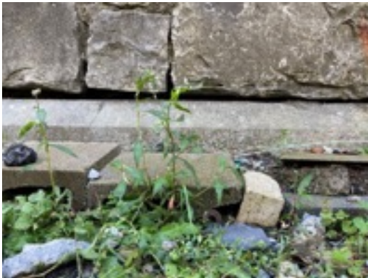
NW Corner of Sanctuary
