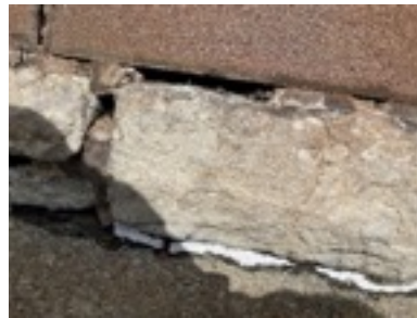
South Wall of Edu Bldg
